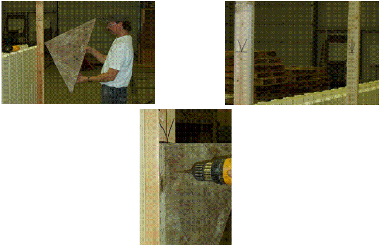
Figure 19: Series of three photographs illustrating placement of scaffold brackets.
