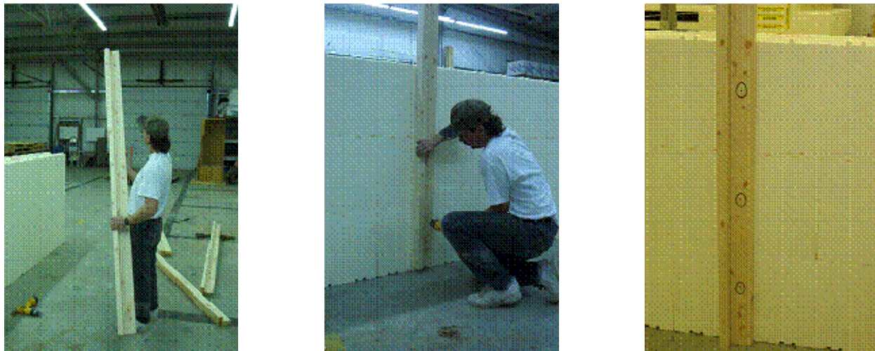
Figure 18: Photographs to illustrate placement of vertical scaffold braces.
