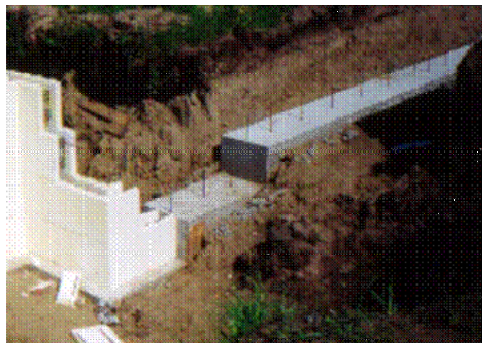
Figure 4: Photograph of Step Footings and Block
